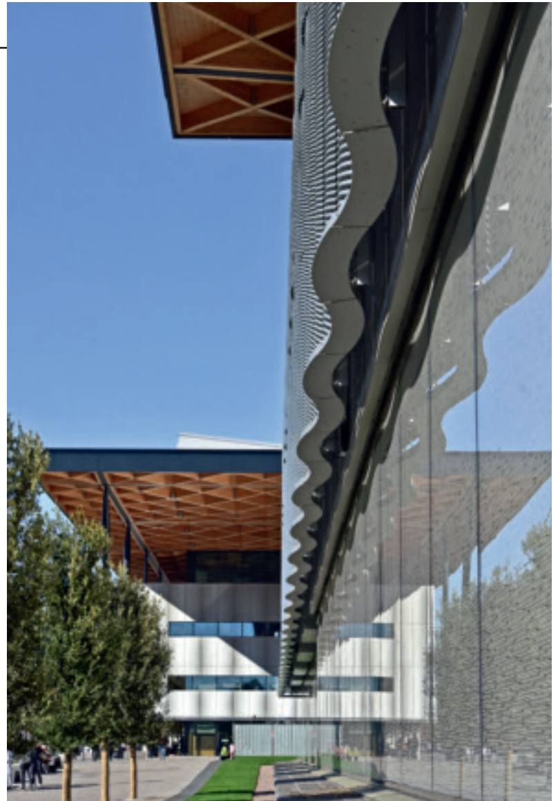
Courtesy of Warwick Manufacturing Group (WMG) – University of Warwick Image courtesy of Paul Scott - Front Elevation
