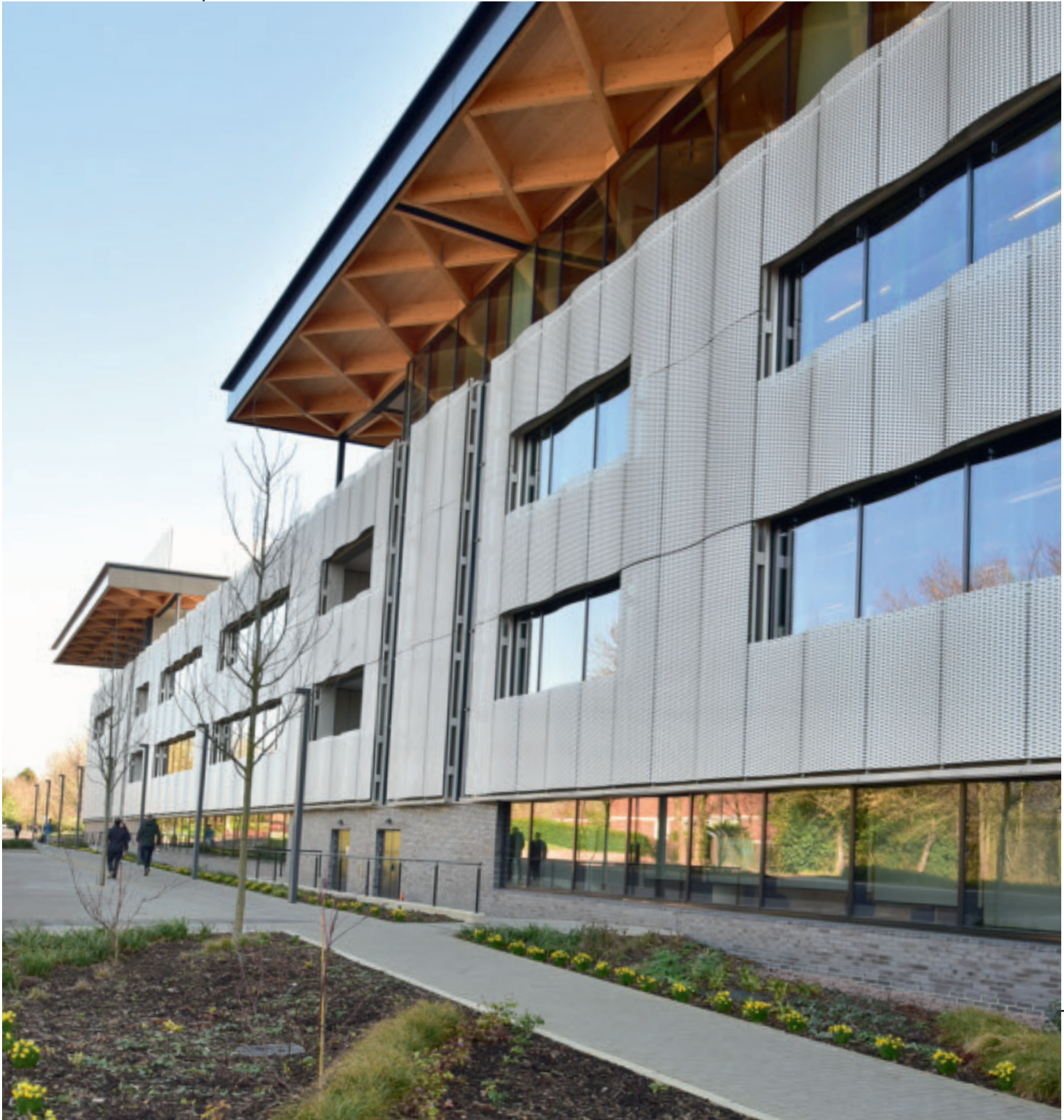
Courtesy of Warwick Manufacturing Group (WMG) – University of Warwick Image courtesy of Paul Scott - Front Elevation
