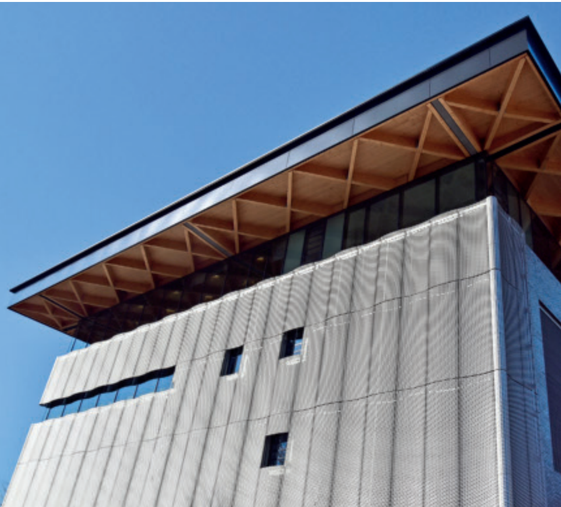
Courtesy of Warwick Manufacturing Group (WMG) – University of Warwick Image courtesy of Paul Scott - Front Elevation
