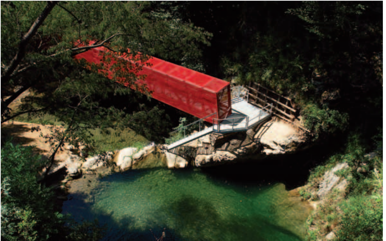
WALKWAY OVER STREAM IN PARCO DEL GIGANTE - BERGAMO (Italy) Design: Arch. Gualtiero Oberti Photo: © Arch. Gualtiero Oberti
