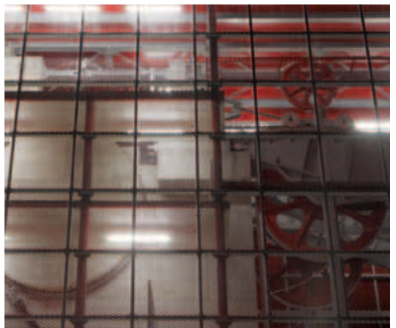
The station enclosure and its utility rooms faced in red lacquered expanded metal ensure ventilation in the rooms while providing protection against the weather and adequate illumination for the boarding platforms at the same time.
