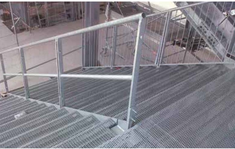
Stair treads for safety stairs
